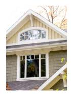
Gables require ornamental elements such as exposed rafters, decorative beams, brackets, louvers, decorative windows, alternate materials or style appropriate architectural detailing. A combination of more than one of such elements is typical of the referenced architectural styles.
